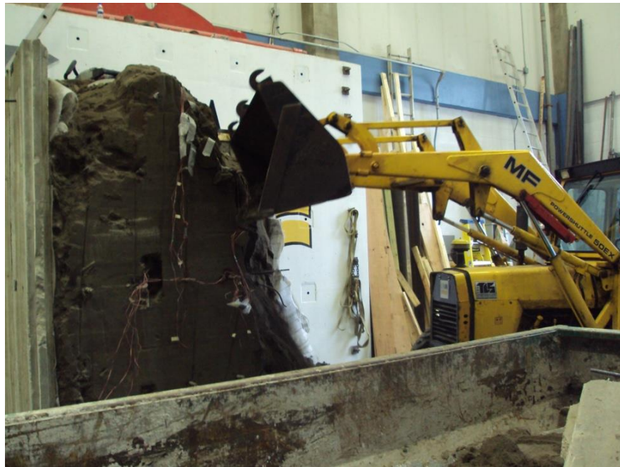
Figure 4.26: (top) Detachment of the panels, (bottom) excavation of CLSM backfill.
